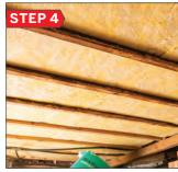
Space StayFast™ brackets 300mm in from each end of the Optimo batt which gives 2 brackets per side per batt.
