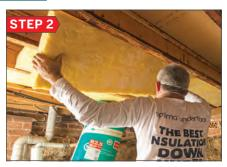
Friction fit Optimo batts tightly between the joists and press in place to ensure there are no gaps between the insulation, underside of floor and joists, or abutting edges (ends) of insulation.
