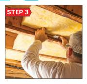
Position Optimo StayFast™ bracket on the side of joist, aligning the bottom of the bracket with the bottom of the joist as shown. Apply pressure to adhere.
