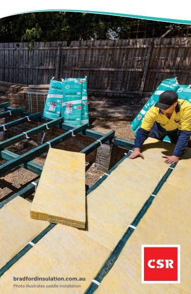
The Building Code of Australia (BCA) requires new homes with suspended floors to be insulated to meet the energy efficiency provisions in part 3.12 of BCA Vol2. The deemed to satisfy requirements are as follows:
